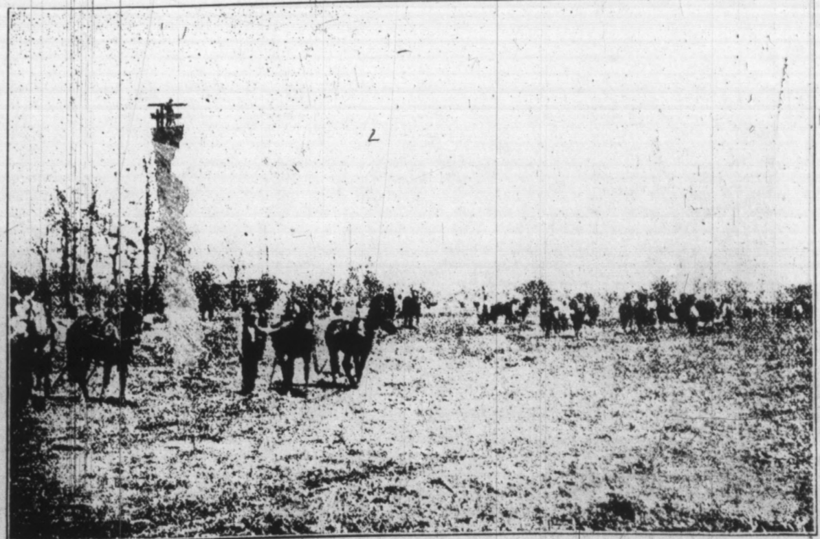
BREAKING GROUND FOR THE NEW RAILROAD SHOPS.
