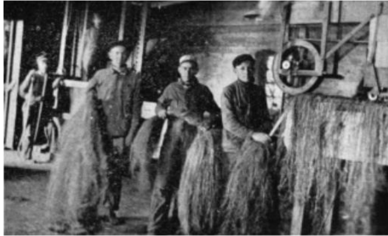
Figure 1.5 Humphrey, J (1919). Long Hemp Fiber as it Comes From the Scutcher Lexington. KY: University Kentucky Agricultural Experiment University Kentucky Agricultural Experiment
