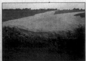
Shown above is a new grass waterway that has been installed on Emily Swift's farm north of Kirksey. An erosion control blanket was placed in the center of Swift's waterway to help stabilize the center until vegetation is established. This practice helps improve water quality by stopping severe gully erosion and filters water before flowing downstream.
