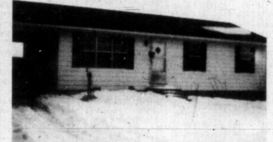
40 ACRES—with 3 bedroom aluminum siding home. Home has living room, one and one-half baths, kitchen with dishwasher, carport, utility room with shower, farrow barn with electricity and water, holds 15 crates, concrete floor, drain system, overhead water systems.
