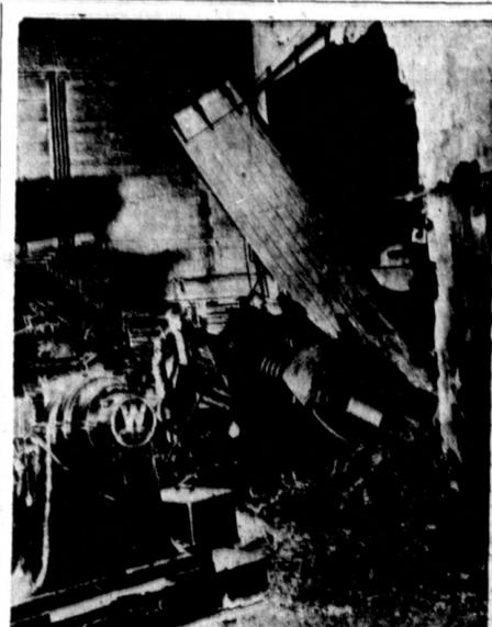
This is what a Pacific Electric Railway substation in Los Angeles, Calif., looked like after a 20-ton armature whirling at 750 r.p.m. tore loose from a generator. One piece of the armature was buried through a six-inch reinforced concrete roof, but no one was injured. Herman Soder, rail employe, examines damage.
