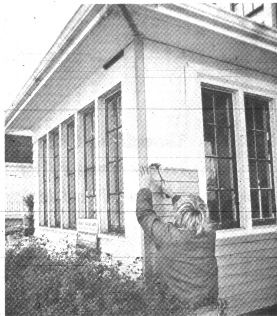
Styrofoam TG brand insulation is a savings dividend for the do-it-yourselfer. Whether it is used in porch conversions, basement remodeling and room additions, over ceilings, sidewalls and masonry walls, or under new siding (shown here), this board-form sheathing product adds the benefits of energy efficiency to any area of the home.
