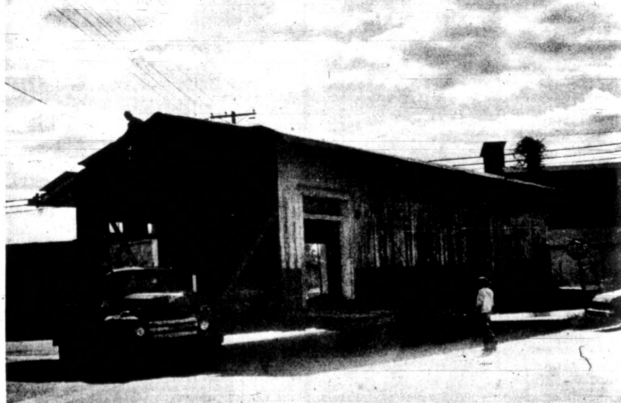
LAST SECTION MOVED — The 45-foot-long third section of the old Louisville and Nashville Railroad depot was moved Friday afternoon completing the relocation process of the depot from Railroad Avenue to the new Murray-Calloway County Park. The movement was delayed somewhat when the section had to be raised a bit to cross a bridge on Industrial Road. Here the depot is shown turning the corner at Main Street and Industrial Road. The last section will be placed in line with the other two next week at the north end of the park near the swimming pool. The structure, which will be renovated by the Murray-Calloway County Community Theatre, will house a park office, headquarters for the Community Theatre, and an indoor area for theatre productions.
