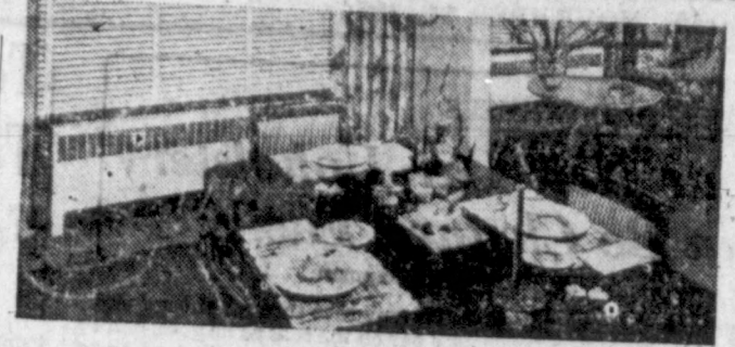
Long, low convactor radiators of modern design, installed beneath the window areas in the living and dining rooms of this modern apartment, supply dependable warmth for cold winter days and blend unobtrusively with the furnishings. Flowered drapes which hang to the floor help frame the modern heating units as well as the window.
