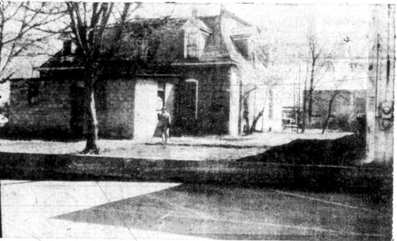
AFTER: This "after" photograph shows Leon standing proudly in the center of the now completely cleaned lot. All the concrete blocks are stacked neatly along the right of the lot and all debris has been raked up and carted away. Mr. Collie cooperated with the Chamber of Commerce in their "Clean-Up, Paint-Up" campaign which is now in progress.
