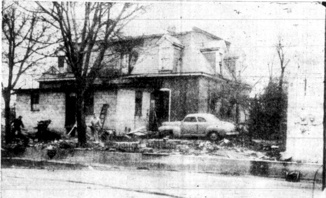
BEFORE: Leon Collie is shown with his two helpers as they begin the task of cleaning up the old T. O. Turner homeplace, located on North Fourth Street and Walnut. As can be seen the entire yard is littered with trash, concrete blocks, and debris.
