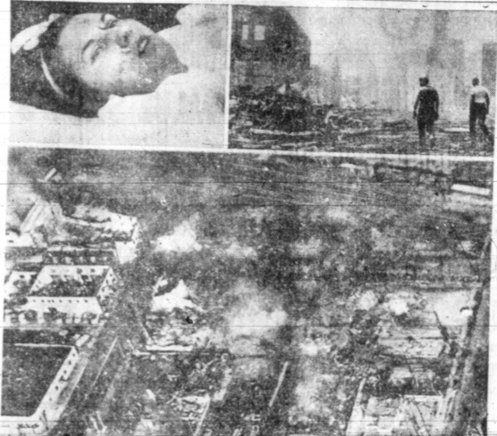
AFTERMATH OF EXPLOSIVES TRUCK BLAST — A parked truck loaded with six and a half tons of dynamite and explosive fertilizer caught fire from a burning building and blew up like a huge bomb in Roseburg, Ore. At least eleven persons were killed and a hundred more were injured, some seriously. Property loss was estimated in the millions. A six-block square area was wrecked and practically every building in the main business district was damaged. At top, left, is Mary-Ellie Unrath, who miraculously escaped with her life. She and a girl friend were on the roof of a house near the center of the blast area when it occurred. At top, right, a youth walks down what was one of the main streets of this city of 13,000 residents. At bottom is an aerial view of the middle of Roseburg, showing the devastation wrought by the explosion. Hole-like a bomb crater, fifty feet in diameter and ten to fifteen feet deep, can be seen in the center.
