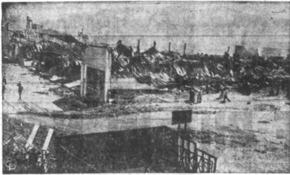
SEARS SEARED DOWN — Bystanders look at smoldering remains of the Sears Roebuck warehouse in Caracas after Communist "commandos" overpowered three guards and set fire to the building. Damages run to $5 million. The burning was a move in a terror campaign against Venezuelan President Romulo Betancourt's Feb. 15 U. S. visit.
