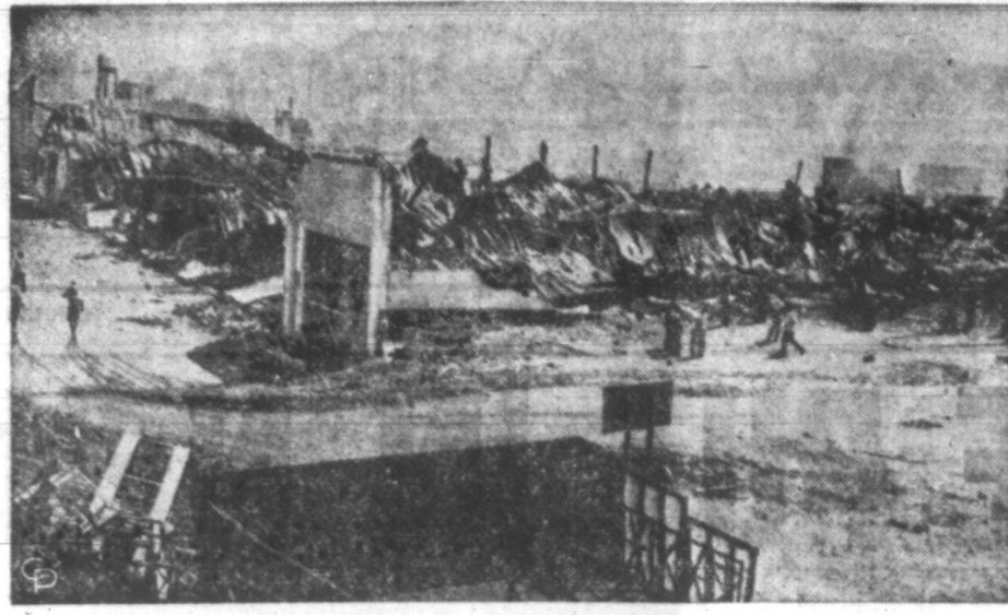
SEARS SEARED DOWN—Bystanders look at smoldering remains of the Sears Roebuck warehouse in Caracas after Communist "commandos" overpowered three guards and set fire to the building. Damages run to $5 million. The burning was a move in a terror campaign against Venezuelan President Romulo Betancourt's Feb. 15 U. S. visit.
