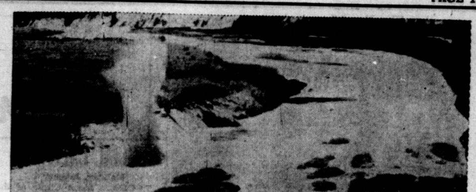
NO DRY RUN, THIS—An explosion of ice and water spews up from the Copper River in Alaska as Navy patrol bombers drop 500-pound bombs to break the ice jam. The ice was backing up water over the Richardson Highway.
