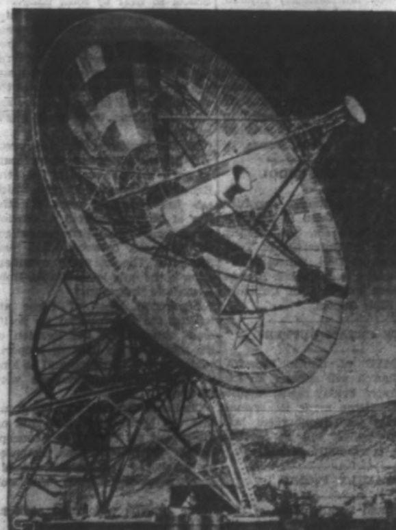
MARS PHOTO RECEPTION—This 85-foot antenna at the Goldstone Deep Space Tracking Station in California is one of the reception points for Mariner-4's photos of Mars. Transmission of a single photo takes eight hours and 35 minutes through those millions and millions of miles of space.
