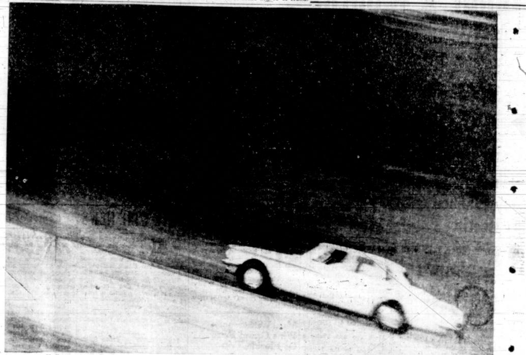
Shell experts test for knock by accelerating up steep grade. In another test, that "fifth wheel" on the back is lowered onto the road to measure mileage precisely.
