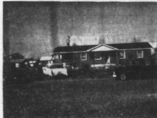
Jerry M. Vaughn is building this nice home on South Ninth Extended. This home has a carport located on one end and is well designed to give comfort, and convenience. There are few vacant lots in the older section of the city and homes are going up every day in the subdivisions located on the edge of the city.
