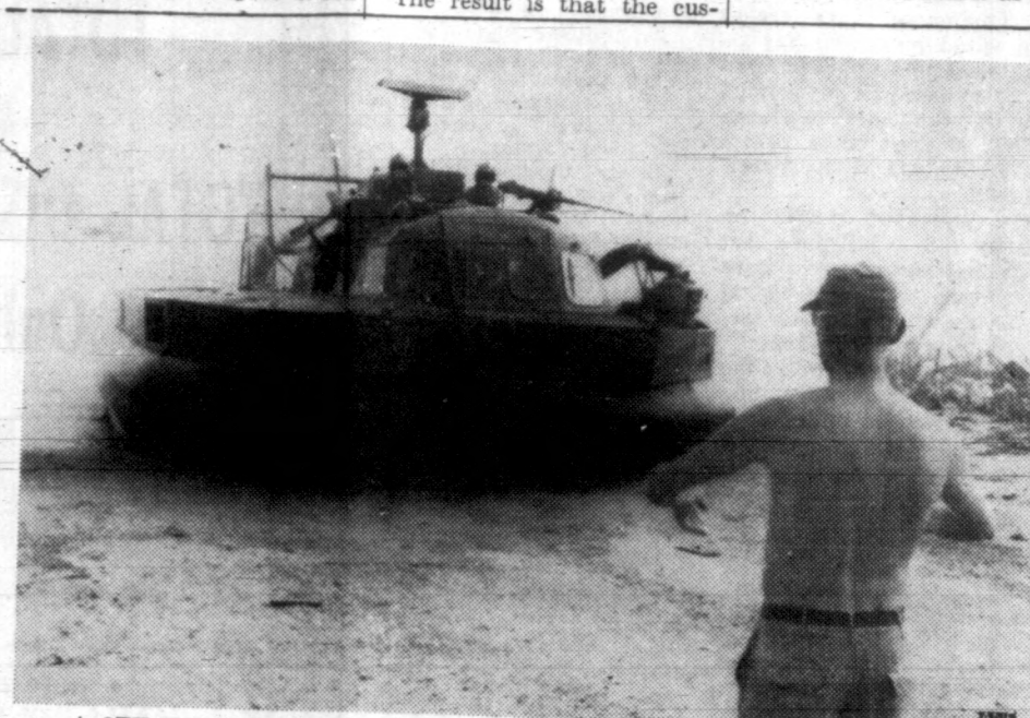
A 9TH INFANTRY DIVISION SOLDIER directs an Air Cushion Vehicle (ACV) ashore after it completed a patrol in the Mekong River Delta region of Vietnam. The ACV, one of three being tested by the U.S. Army in Vietnam, is built by Bell Aircraft Corp. of Buffalo, N.Y. The ACV is armed with two .50 caliber machineguns mounted in twin turrets atop the cabin, two M-60 machineguns mounted on either side of the boat and a 40mm grenade launcher on the port bow. The hard bottom of the craft is supported on a four foot cushion of air, enabling it to travel over land, water, mud or marsh.
