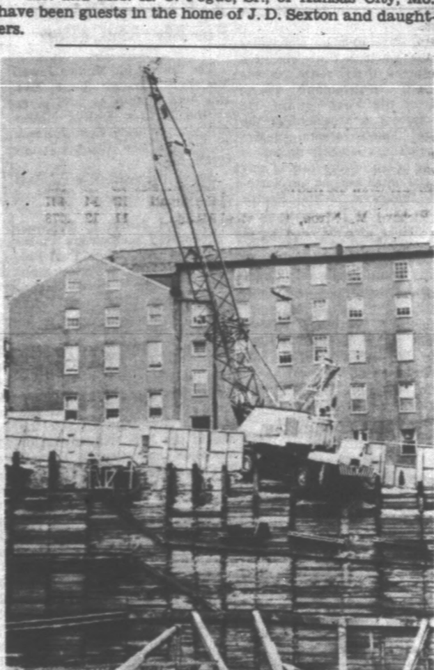
IT WAS THE CRANE'S NECK, ALMOST—A 140-ton crane balances partly over the edge of a 40-foot drop at a construction excavation in downtown Baltimore. Police suspect sabotage of the $287,000 tool, since the steering wheel was lashed with rope. That boom reaches 120 feet high.
