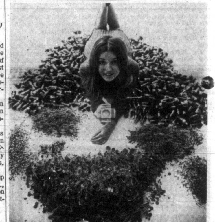
ONE REPLACES 6,200 - A model holds a Texas Instruments electronic circuit, called an LSI (large scale integration), that replaces all those items around her - 4,000 transistors, 1,500 diodes, 700 vacuum tubes - used in electronic equipment.
