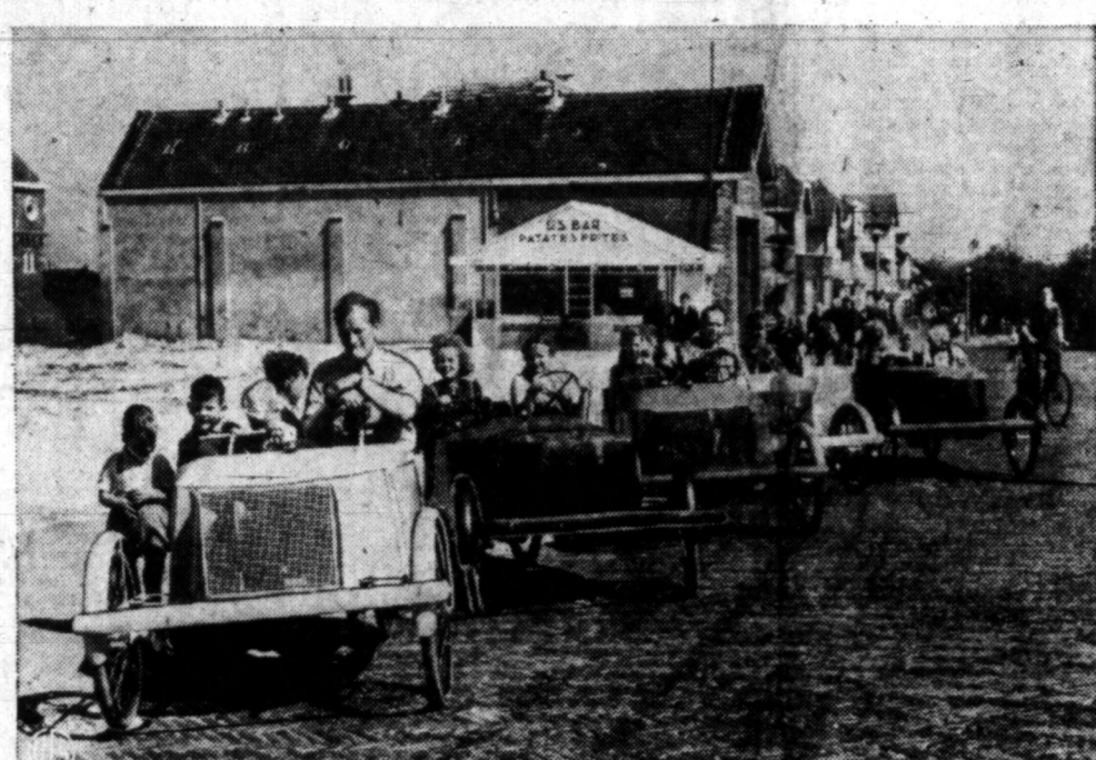
FOOT POWER MOVES DUTCH TAXIS —Gasless cars called "Fietstaxis," which accommodate three adults, have made their debut at Zandvoort-by-the-Sea, Holland. If you don't mind pedaling you can get a nice breezy ride. Made of lightweight metal and using bicycle-type wheels, there is one control for steering and a set of double pedals for motive power.
