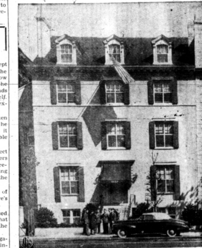
TEMPORARY "WHITE HOUSE" —President Truman and his family will move from the White House, termed a "fire trap," to the Blair House soon after Mr. Truman returns from his Florida vacation so that repair work can begin. Here is the street-view of Blair House, which has been used as a residence for visiting foreign dignitaries.
